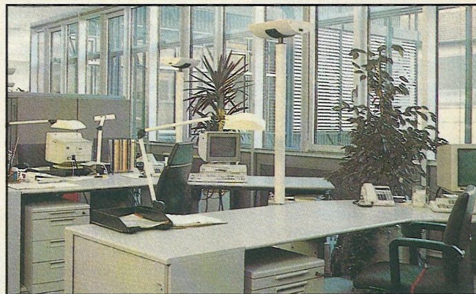
The Waldmann office lighting system uses screen mounted luminaires for ambient lighting.
